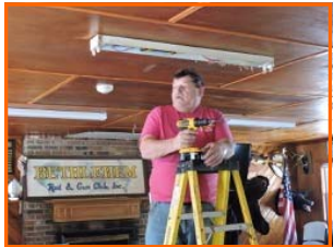
New fluorescent lighting in clubhouse
